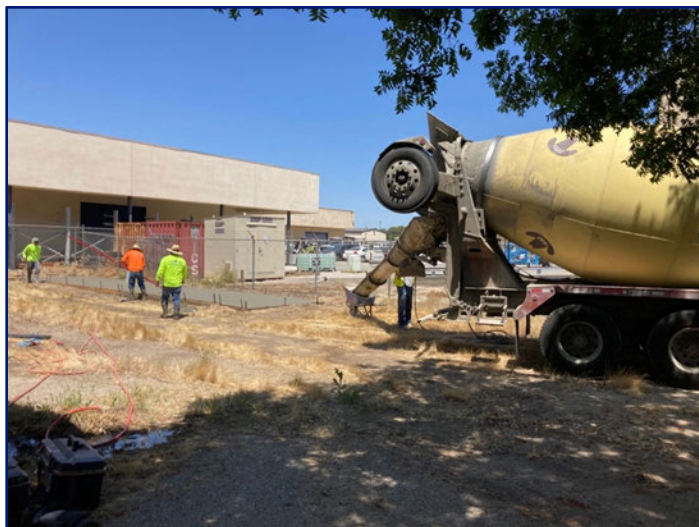
A concrete pad is poured next to the CWSR for a new container full of well data and samples from Long Beach.
